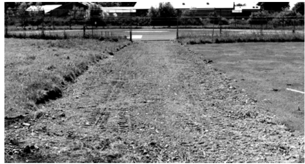
The new line park after gravel topping
